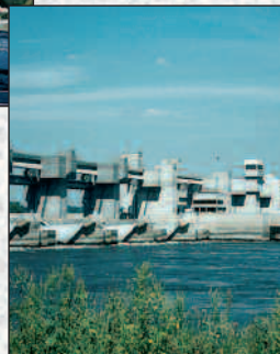
Lock and Dam
